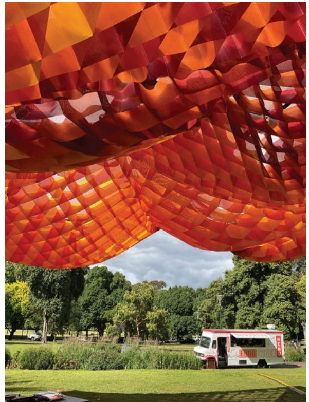
Figure 5.28 The 2022 MPavilion is made up of fabric and tensile architecture with the outermost layer made from fishing nets, which creates the tactile texture. The fabric roof is a reminder of making things with our hands such as traditional fishing nets, while the space underneath creates an open space that is used for many community activities, including ‘making’.
