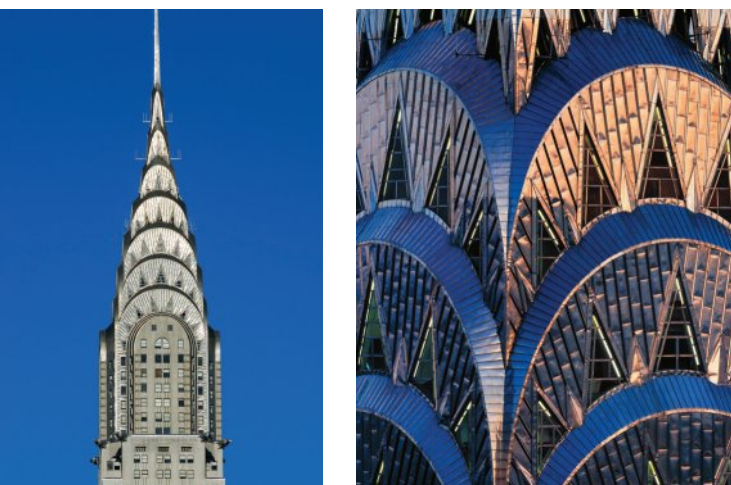
Figure 5.9 The Chrysler Building, New York City, is an example of Art Deco
