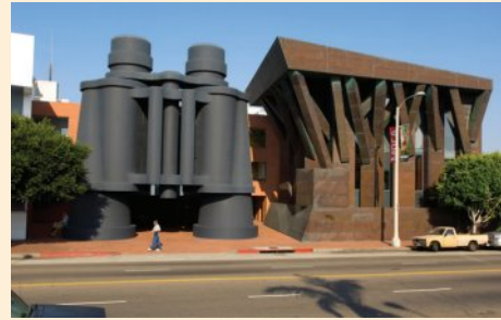
Figure 5.26 Giant binoculars in front of building designed by architect Frank Gehry in Venice Beach, California, USA
