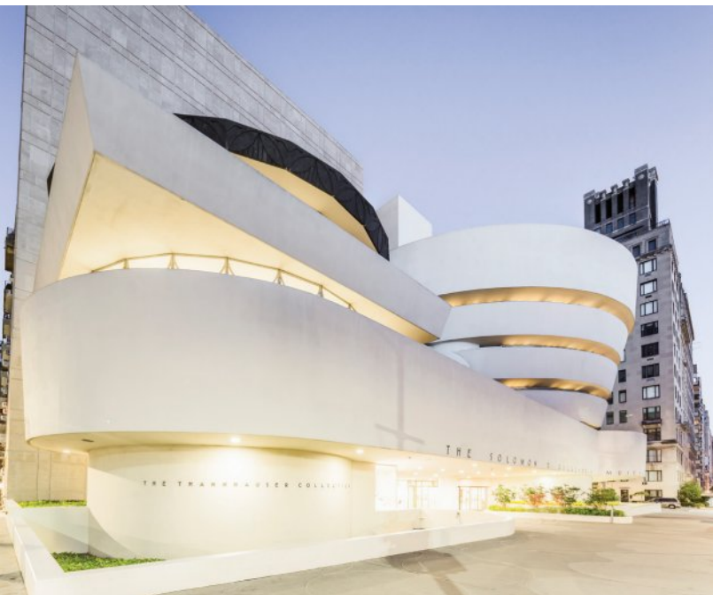
Figure 5.6 Exterior view of Guggenheim Museum by Frank Lloyd Wright. Aiming to break away from the traditional museum layout, which forced visitors to progress from space to space and then back through to exit, Wright designed the gallery as a continuous ramp.
