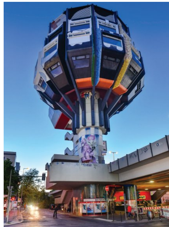
Figure 5.20 Beer Brush Tower, Pop-Art futuristic building designed by architects Ralf Schüler and Ursulina Schüler-Witte, Berlin
