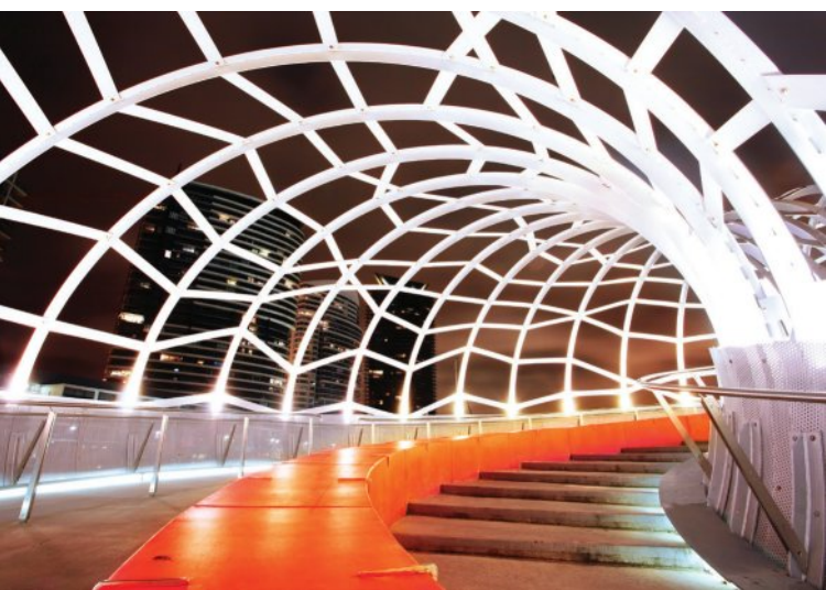
Figure 3.33 Webb Bridge in Melbourne's Docklands
